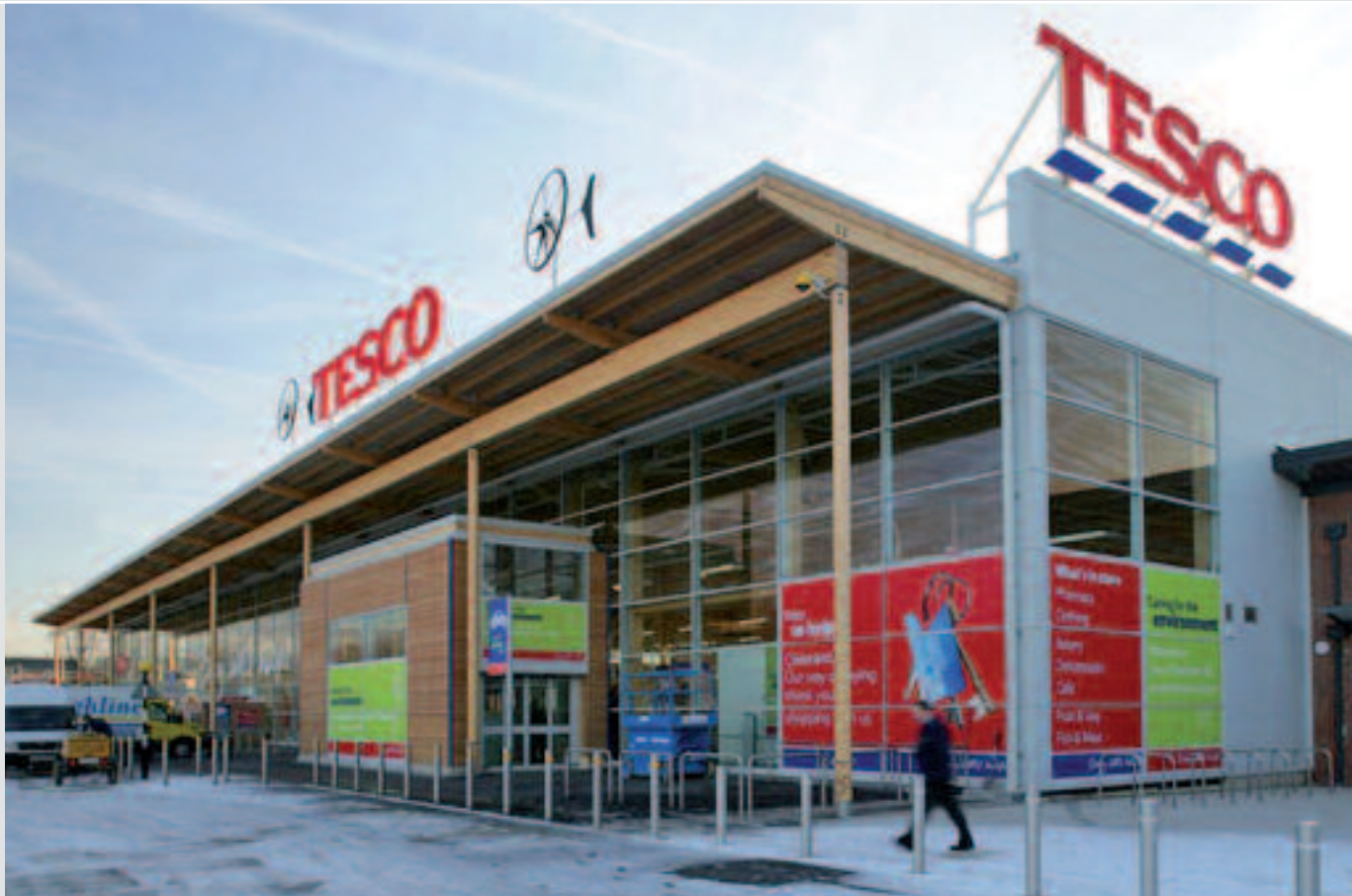
Photo credits: B&K Structures
