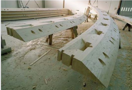
Glulam beam after final CNC-processing
