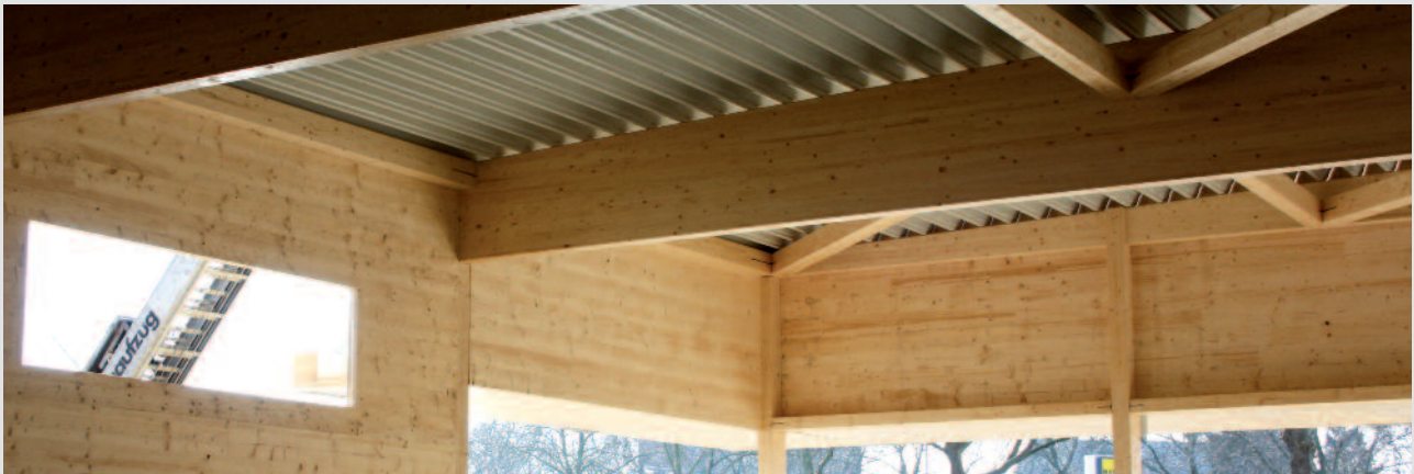
Rapid roofing will provide the best protection of visible surfaces from weathering effects.
